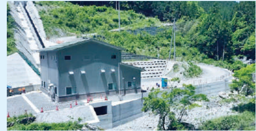
Kurofujigawa Power Plant (Kumakogen Town, Ehime Prefecture)
