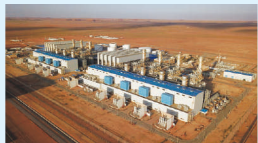
Power generation output 1,730 MW (owned capacity 220 MW)
