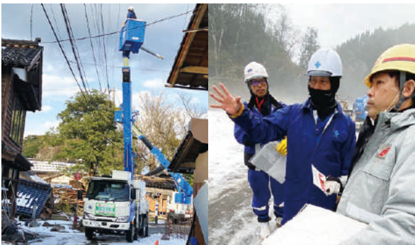
Support for recovery operations following the Noto Peninsula earthquake (Early dispatch of a total of 126 personnel with aerial work platforms, etc.)
