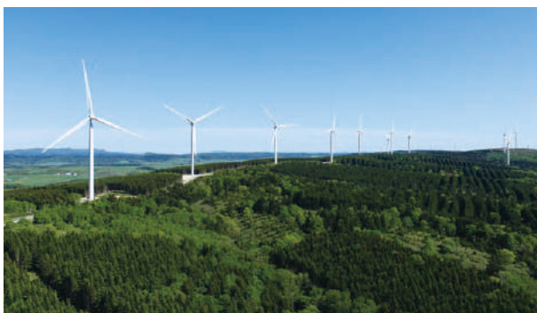
Example construction from Yonden Engineering Co., Inc. (Kawaminami Wind Farm, Hokkaido)
