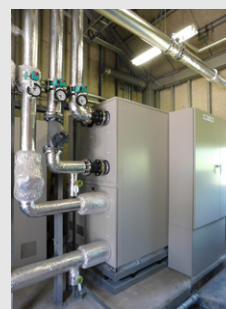
Heat-pump hot air generator
