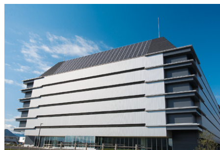
“Powerico” data center in Takamatsu
