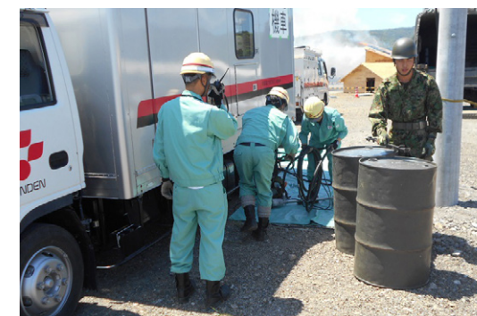
Fueling of high-voltage power generator
