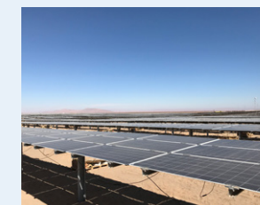
Installation of more than 300,000 solar panels
