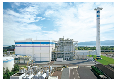
Replaced with highly efficient LNG combined cycle system (Sakaide Unit No. 2)
