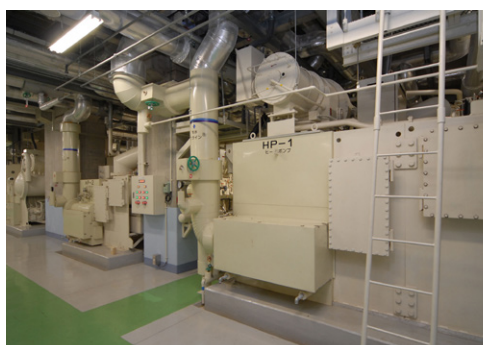
Exhaust heat recovering heat pump (machine room)
