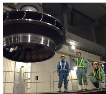
High-efficiency turbine runners at Bunsui Daiichi Power Station
