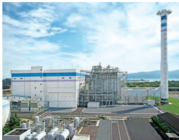
Replaced with highly efficient LNG combined cycle system (Sakaide Unit No. 2)
