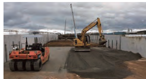
Construction work on a state road using "Porous Sand" soil conditioner, a lightweight embankment material (Tokushima Prefecture)
