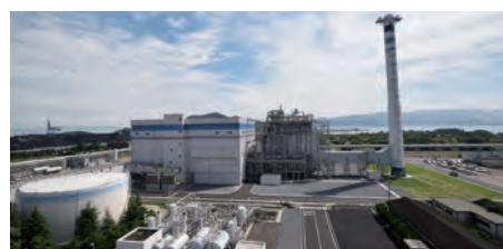
Replaced with highly efficient LNG combined cycle system (Sakaide Power Station Unit No. 2)
