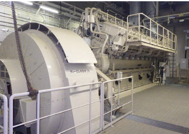
Emergency diesel generator used for online maintenance demonstration
