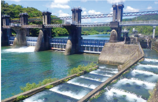
Example of fishway installation: Saga Intake Weir (Saga Power Station)
