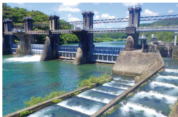
Example of fishway installation: Saga Intake Weir (Saga Power Station)
